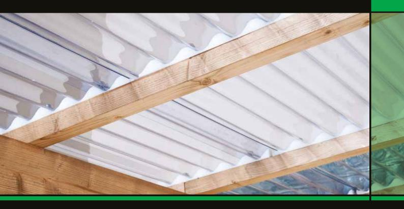
Corrugated PVC Sheets combines low weight with strength, durability with aesthetics and offers a cost-effective solution for both Commercial and DIY applications.
